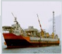
2000 Asgard A&B FPSO & Hull • Norway • 16000T Topside
